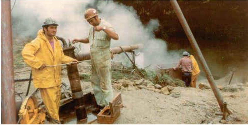
Geothermal well at S. Pedro do Sul
