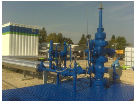
Closed-loop geothermal well „Prottes T11“ near Vienna (thermal capacity ~ 200 kW) © OMV, 2009
