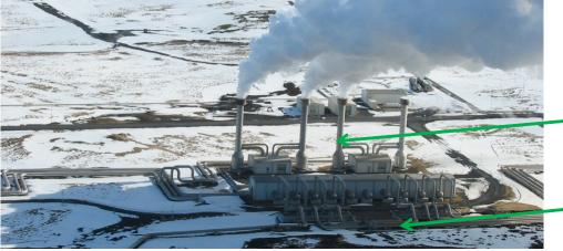
Production Two phase Well flow Steam vent station Separation station
