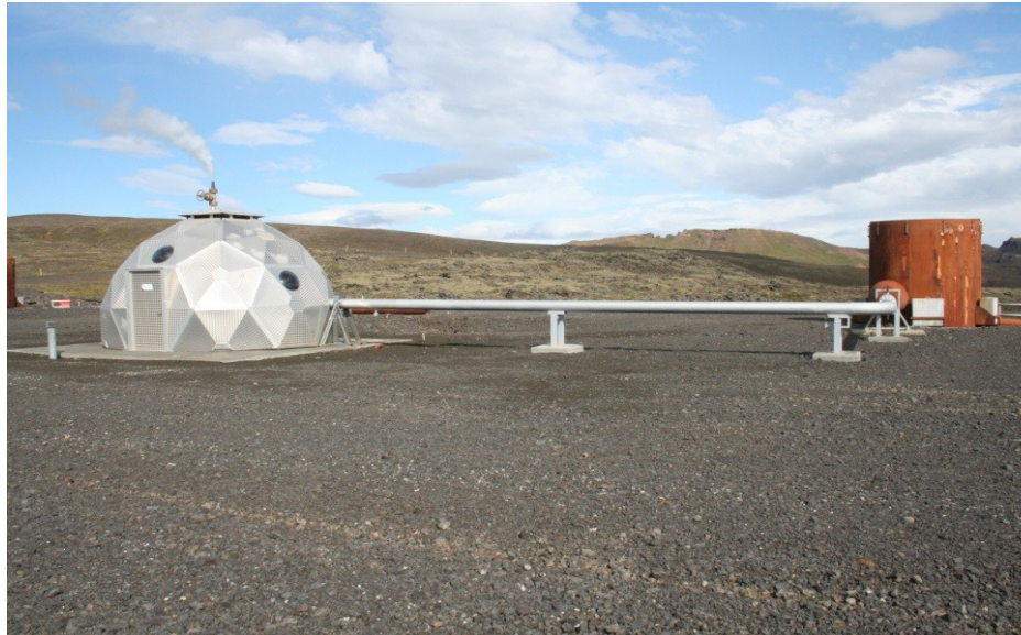
Enclosed wellhead connected to a muffler
